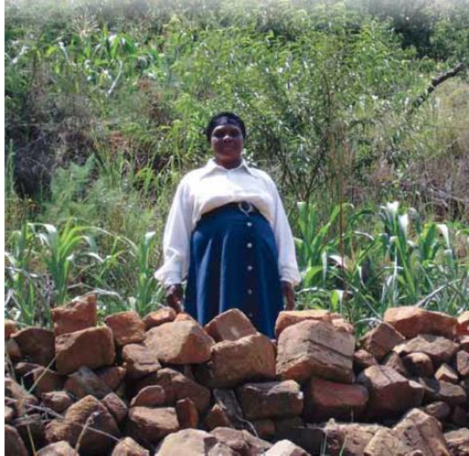
Picture 1: Stone terrace for retaining rainwater and soil
